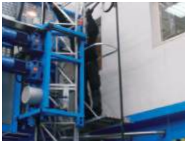
Auxiliary catwalk for anchorage assembly
